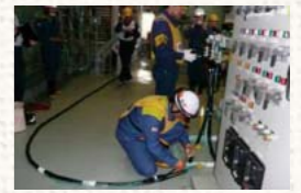
Conducting a drill to connect equipment to a vehicle-mounted generator
