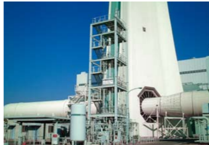
●CO 2 recovery pilot plant at Nanko Power Station
