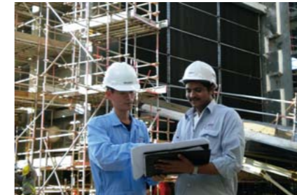
●Repowering work at the Senoko Power Station
