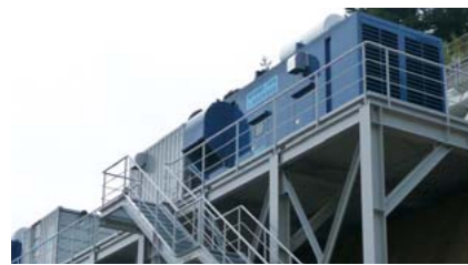
● Air cooling emergency power generators
