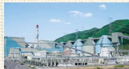
Operation at Maizuru Power Station was swiftly restored
