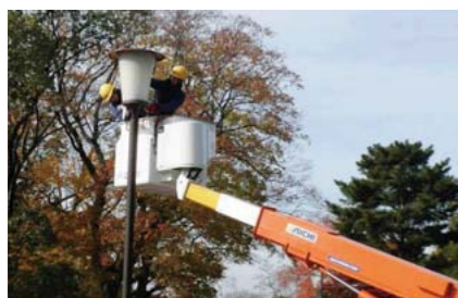
●Using an aerial work truck to clean streetlights (Nara)
