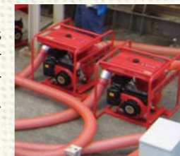
A total of 70 engine-driven seawater pumps were installed at our nuclear power plants
