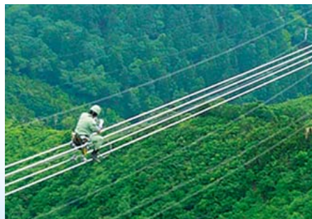
● Maintenance of transmission lines
