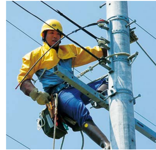
●Distribution line maintenance
