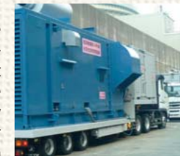
A total of 21 air cooling emergency power generators have been installed on elevated ground at our nuclear power plants
