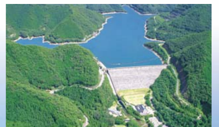
● Tataragi Dam at the Okutataragi Power Station
