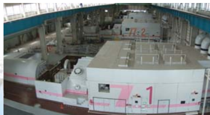
● Combined-cycle power plant (Sakaiko Power Station)
