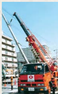
Recovery work after the Hanshin-Awaji Earthquake
