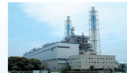
● Himeji No. 2 Power Station in its current state
