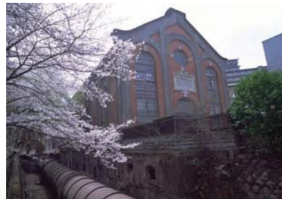
● Keage Power Station (former building) and a penstock
