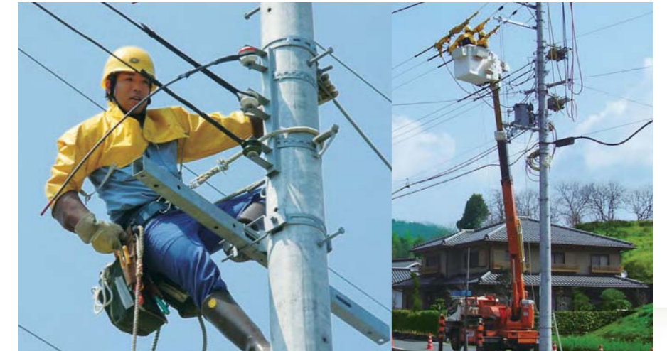
●Distribution line maintenance
