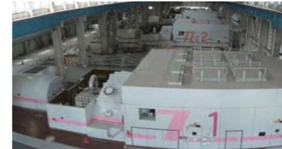
● Combined-cycle power generation equipment (Sakaiko Power Station)
