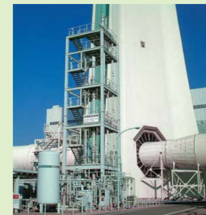
●Flue gas decarbonization plant at Nanko Power Station
