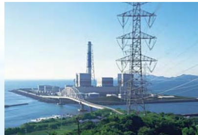
● The Gobo Power Station
