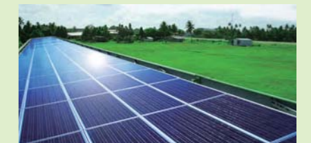
●Solar power generation equipment set up on a soccer field
