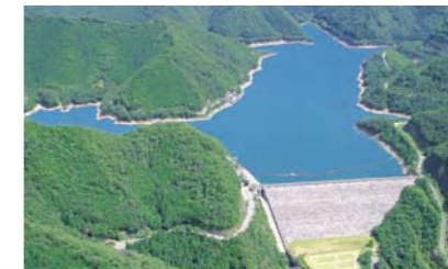
● Tataragi Dam at the Okutataragi Power Station
