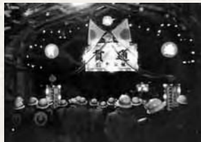
In February 1958, the most difficult part of the Kurobegawa No. 4 project, the Kanden Tunnel, was completed.
