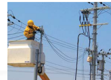
●Distribution line maintenance
