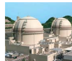
● Ohi Power Plant
