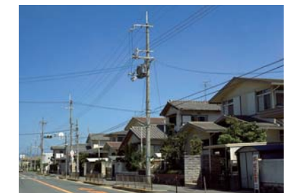
●Electrical pole and transformer
