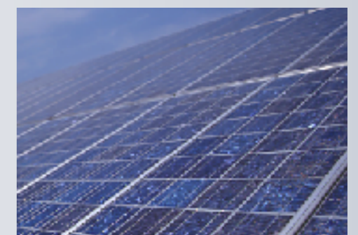
Solar panels ( Nanko Thermal Power Plant )
