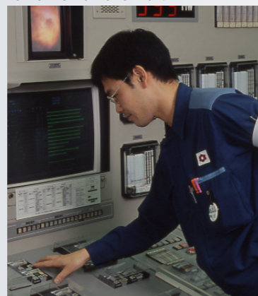
Nanko Thermal Power Plant
