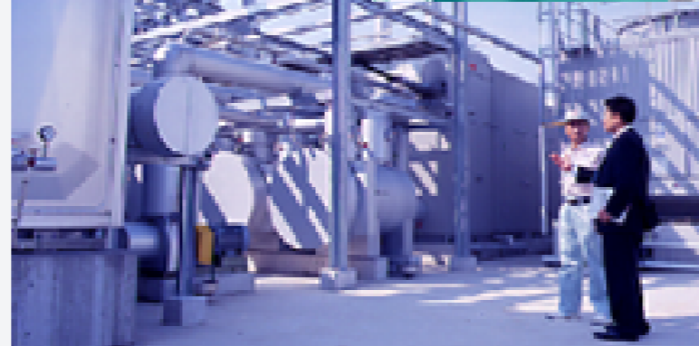
"Eco Ice" thermal storage system
