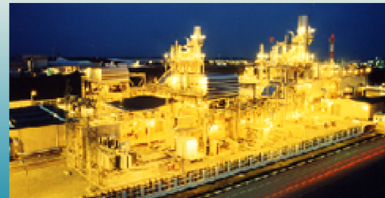
Thailand's Rojana Power Co., Ltd.
