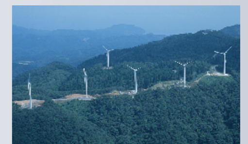
Wind-power generation equipment supported by the Kansai Green Power Fund (Taiko-yama, Kyoto)
