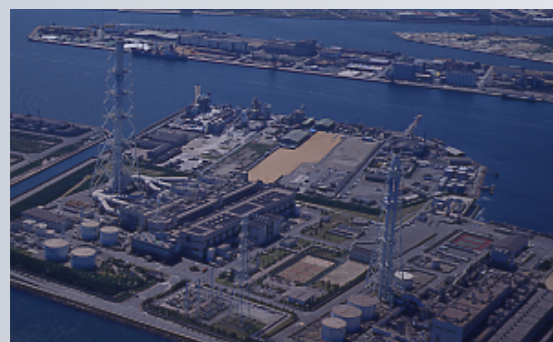
Himeji No.1 Thermal Power Plant
