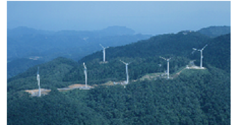
Wind-power generation equipment supported by the Kansai Green Power Fund (Taiko-yama, Kyoto)
