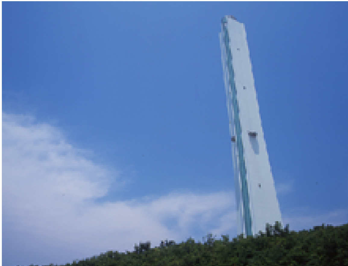
Nanko Power Plant (ISO14001 certified)
