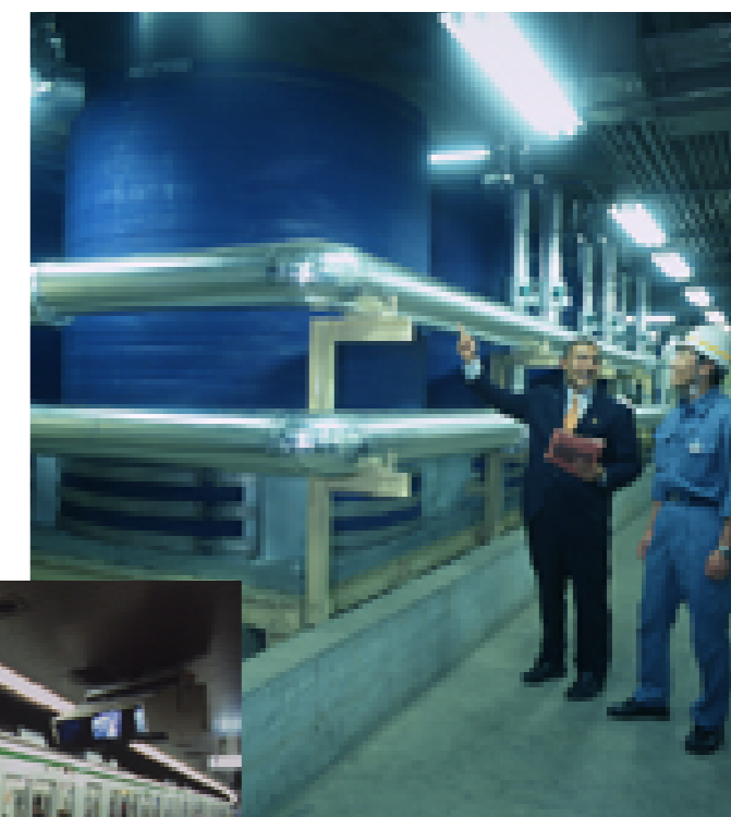
"Eco Ice" thermal storage system
