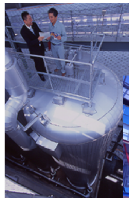
"Eco Ice" thermal storage system
