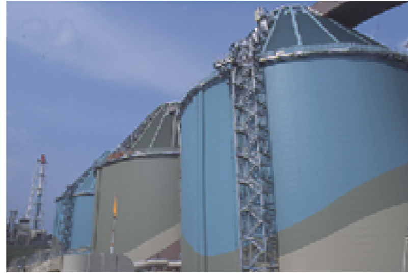
Maizuru Thermal Power Plant
