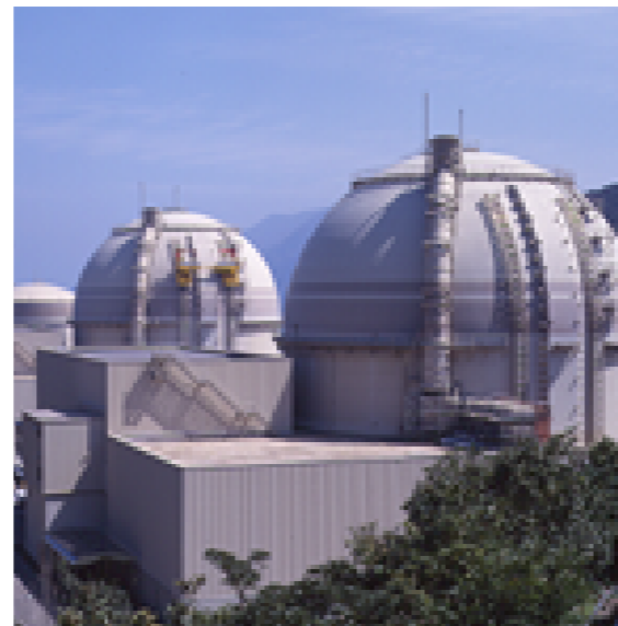
Ohi Nuclear Power Plant (4,710 MW)
