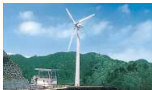
Wind-energy generating equipment at Okutataragi Pumped-storage Plant.
