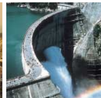
Kurobegawa No.4 Hydro Power Plant.
