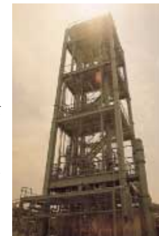
Flue-gas decarbonization pilot plant set up within Nanko Power Plant. Research is under way into recovery of CO 2 present in power-plant flue-gas emissions.
