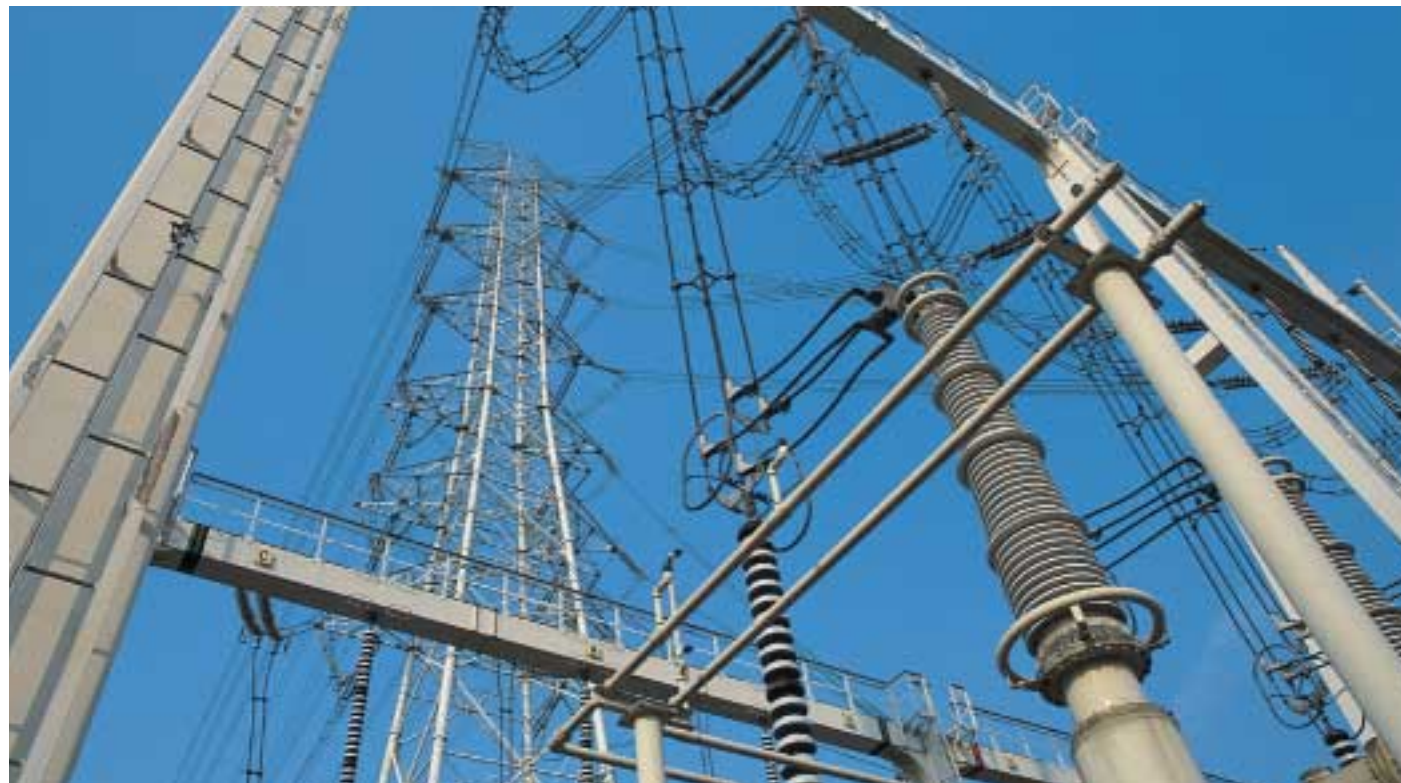
Special high-voltage transmission installation. 500 kV pylon.
