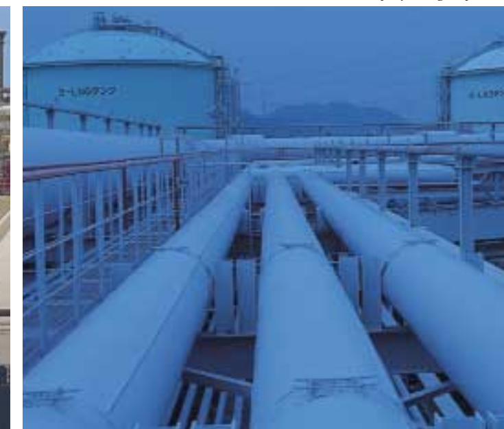
LNG base at Himeji No.2 Power Plant. It serves as the base for companywide gas operations.
