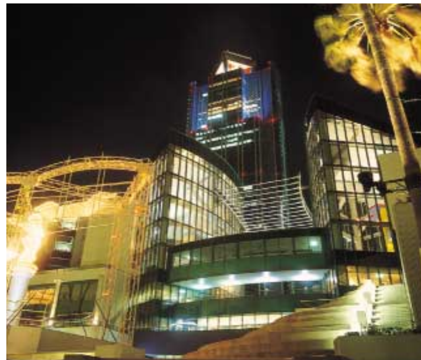
The Asia and Pacific Trade Center (ATC)/ The Osaka World Trade Center (WTC). An office and commercial complex located in the Nanko district of Osaka.
