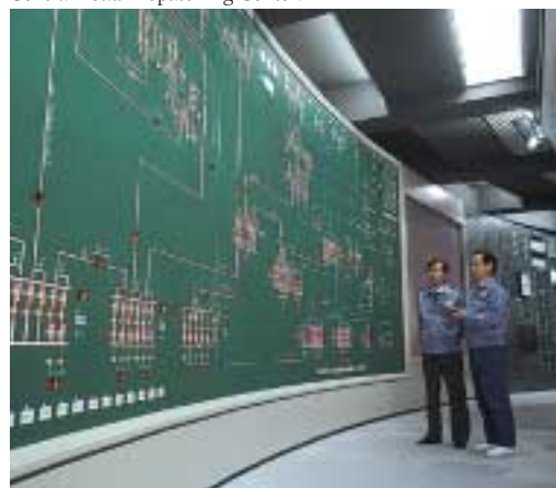
Central Load Dispatching Center.
