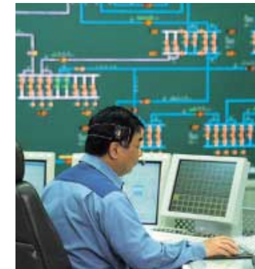
Central Load Dispatching Center. Power supply status throughout the company's network is monitored 24 hours a day.
